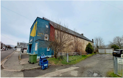
Former cinema building.
