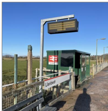
Figure C4: Llanbedr Railway Station
