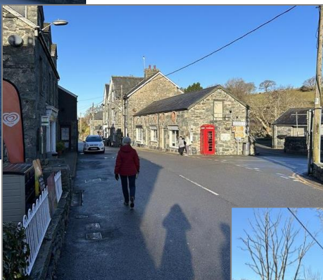
Figure C7: Pedestrians required to walk on the road due to lack of footways.
