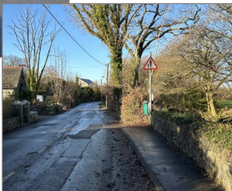
Figure C8: Footway along Mochras Road ends abruptly
