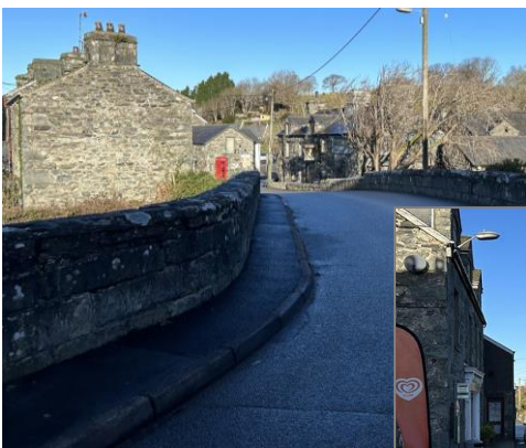
Figure C6: Narrow footway across the Afon Artro bridge
